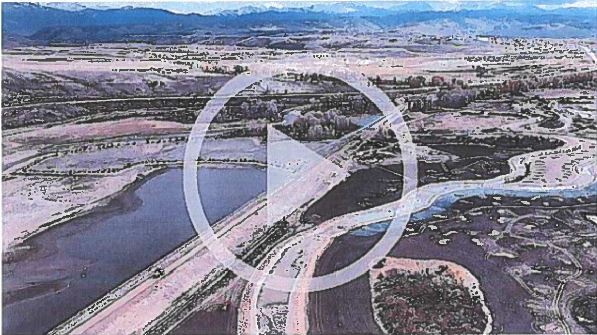
Water has started to flow in the Colorado River Connectivity Channel near Windy Gap Reservoir in Grand County.
