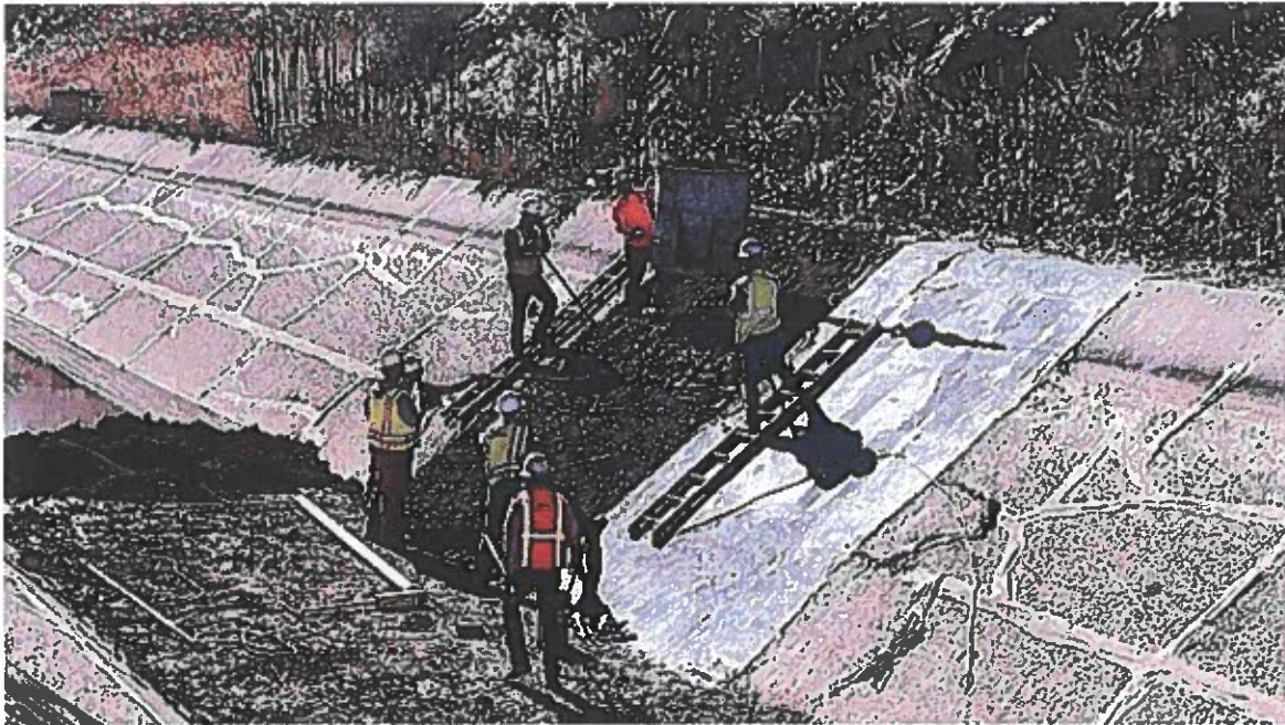
Crews replace concrete panels along the Charles Hansen Feeder Canal.
