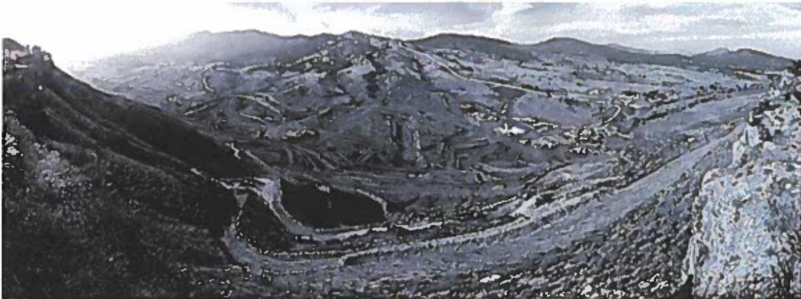
Panoramic view of the work at Chimney Hollow Reservoir on Nov. 9, 2021.
