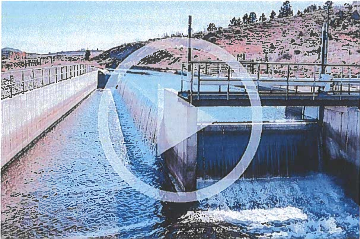
Preparation to ensure the C-BT Project is ready for water deliveries takes a lot of work.
