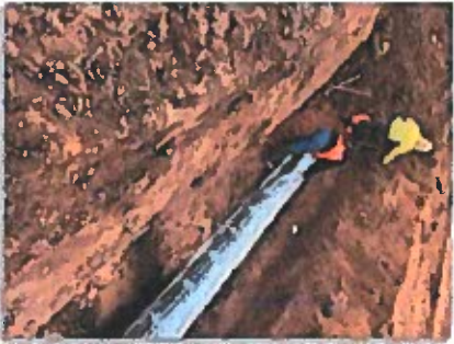
painted ready for backfill at 255.jpg
