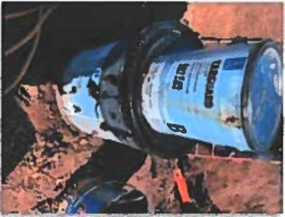
apply seams on half inch over lap.jpg
