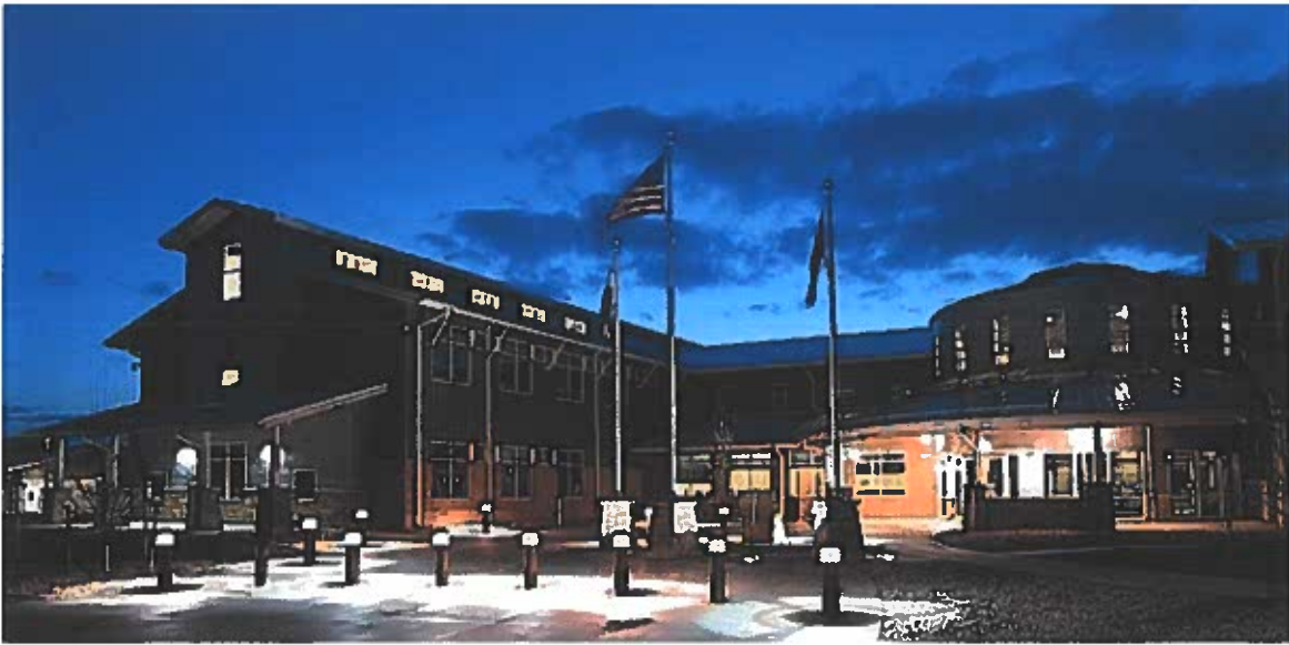
Northern Water's headquarters are in Berthoud, Colorado.
